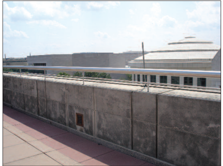
A permanent guardrail and parapet protects a rooftop terrace.
