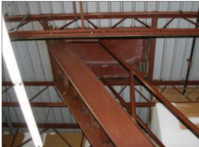
Ships ladder access to roof hatch
