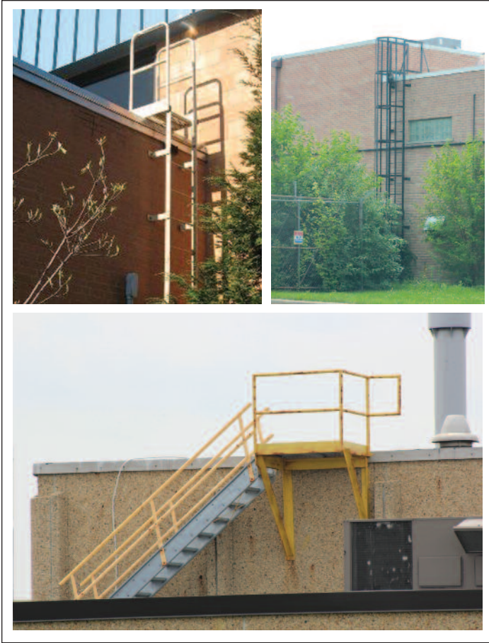
Exterior staircase and fixed ladders for roof access
