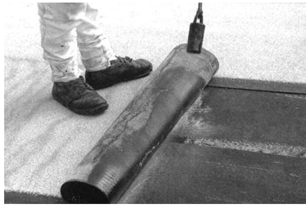
Photo 2: A roofing worker is advancing a roll of membrane.
