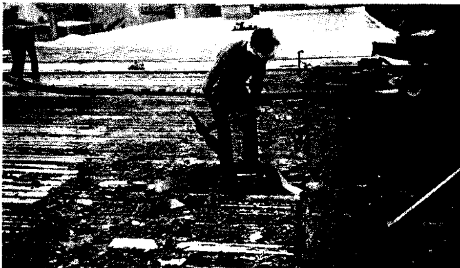
Roof tear-off in progress
