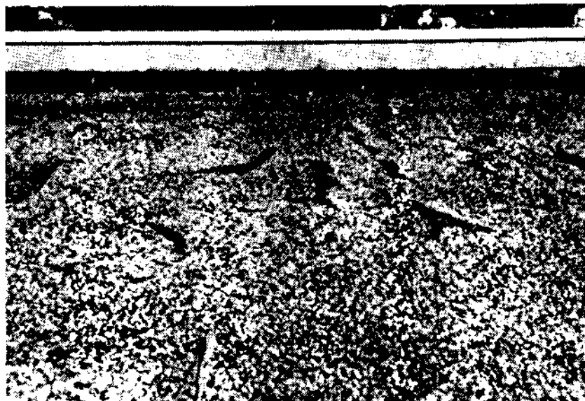
Small buckles in roof membrane
