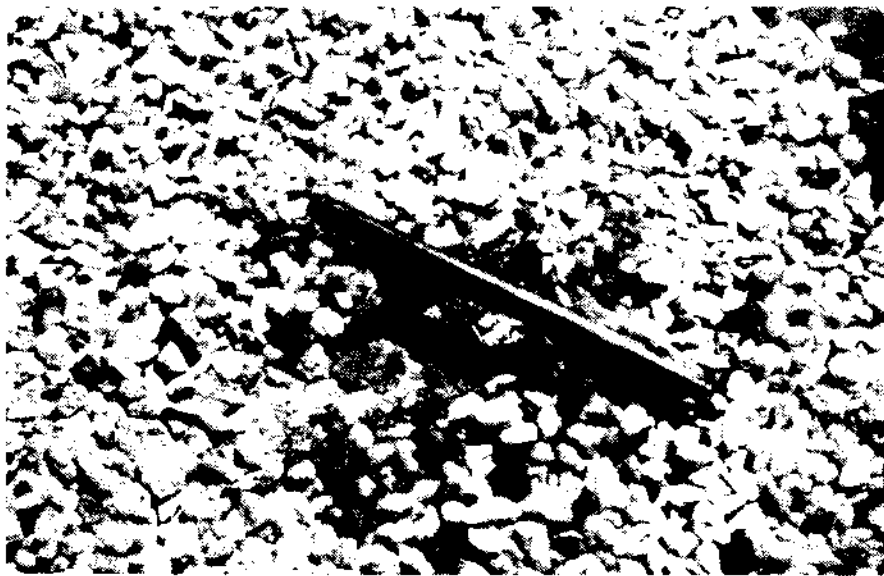
Puncture in roof membrane from dropped tool
