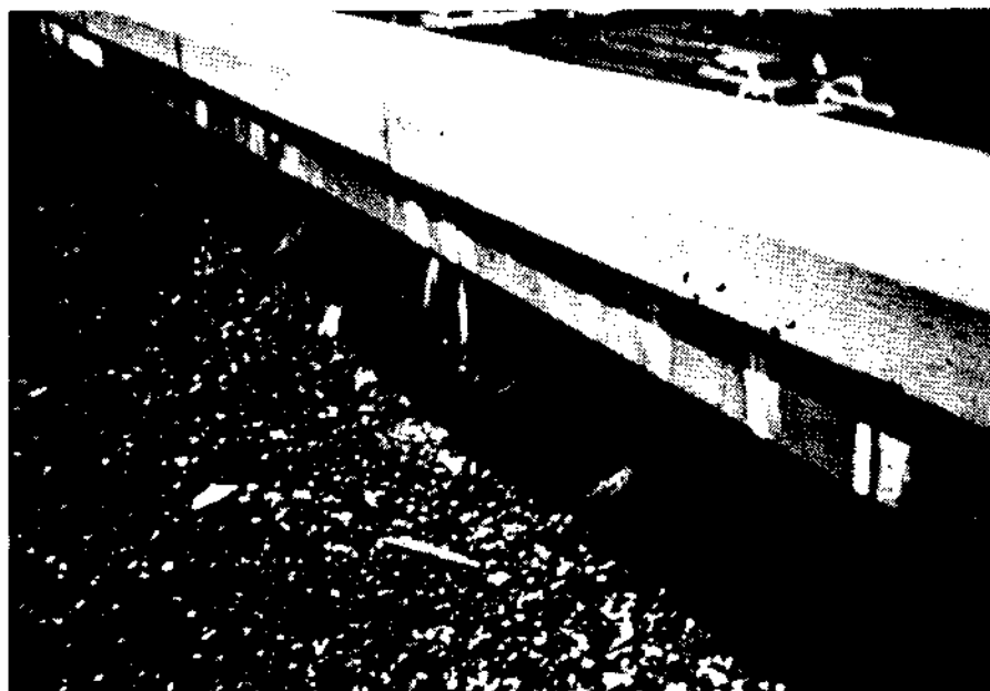
Wrinkled base flashing at parapet wall
