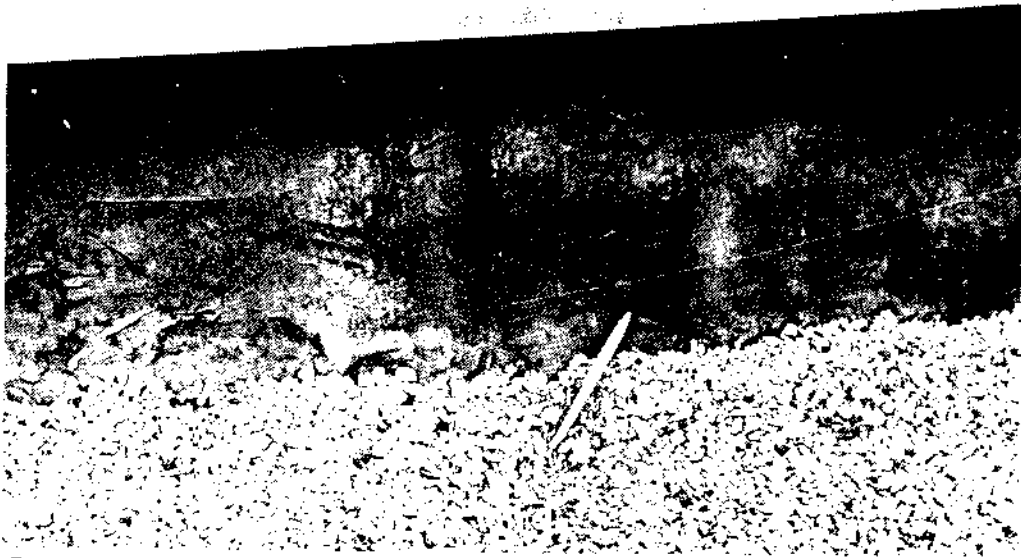
Puncture at bottom of base flashing
