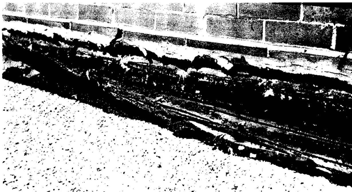
Base flashing separated from parapet wall
