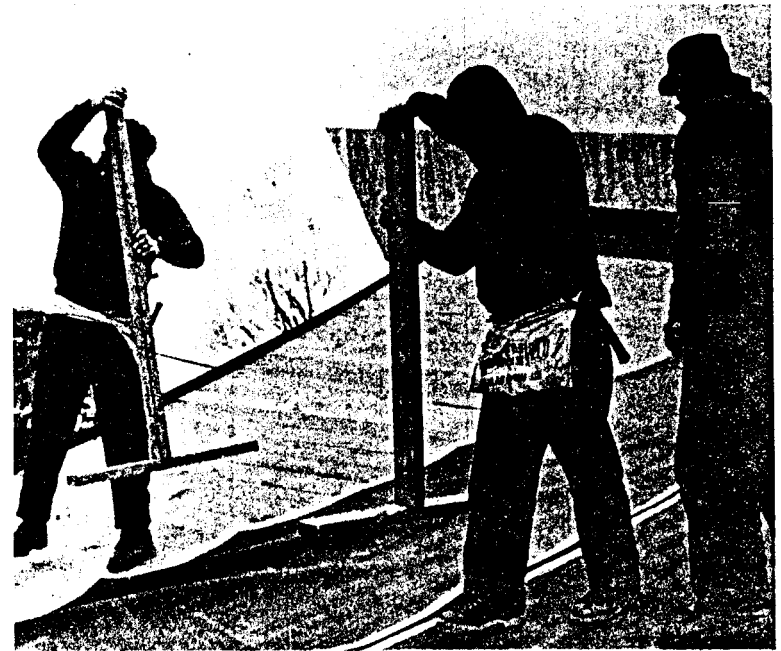
Workmen tap down the aluminum strips attached to the edges of the neoprene sheets used on the Ingalls Hockey Arena roof.
