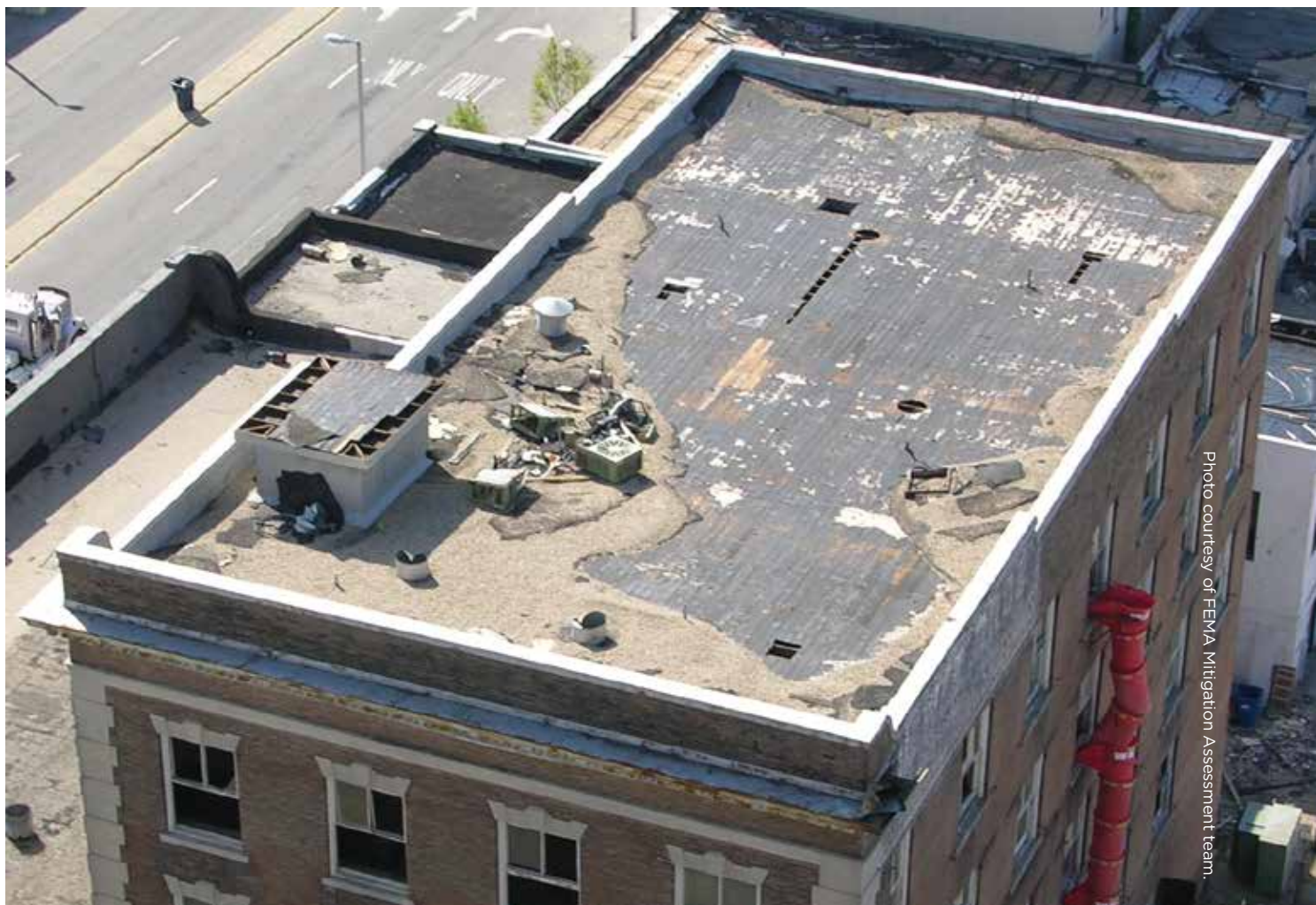
Photo 2: Most of the aggregate and insulation blew off this built-up roof system. The damaged membrane cannot be repositioned; a permanent or new temporary roof is needed to provide watertight protection.
