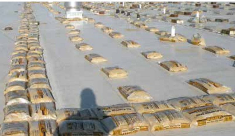
Photo 5: This double row of sandbags occurs at the interface between adhered and unadhered areas.
