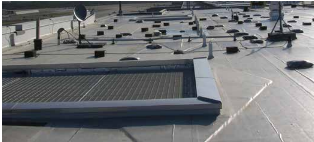
Photo 4: Emergency ballast was installed after a single-ply membrane detached from the insulation.
