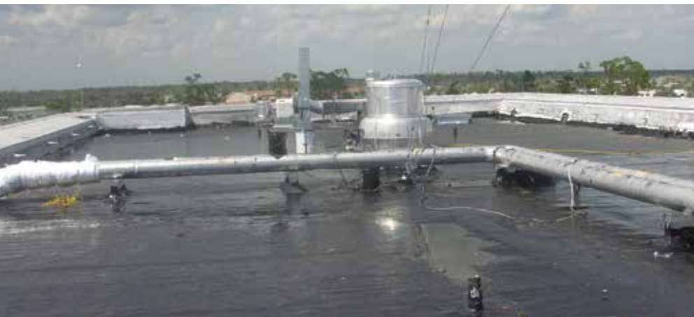
Photo 3: This building's roof was temporarily secured with a two-ply built-up roof. (Photo courtesy of FEMA MAT, Hurricane Charlie 2004.)
