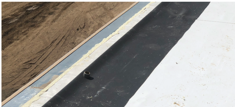
Photo 3: A view of a roof perimeter near completion. Note the spray foam at the roof edge between the insulated metal panel wall and the insulation and cover board, sealing against air movement. Additionally, a strip of butyl with its release paper still in place is installed and ready at the outside edge of the galvanized insulated metal panel wall cap.
