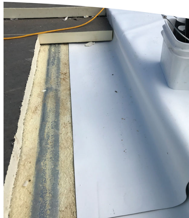
Photo 1: A field installation of an air-stop detail between a loading dock at 55 F and a food-production area at 36 F. Note the deck flutes are filled solid and the membrane has been dropped to the deck to prevent air movement between the areas.
