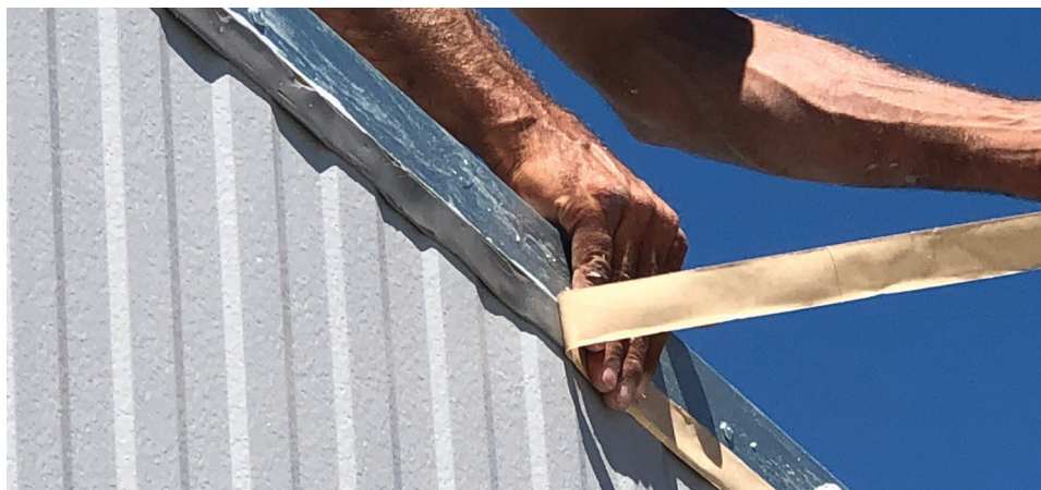
Photo 4: A view of a worker removing the release paper from a butyl strip on the exterior face of an insulated metal panel wall. This is the primary air seal. After the membrane is flopped over the wall, a heavy-gauge metal cleat will be fastened through this butyl strip. This will provide a compression seal as well as the cleat for the edge metal. Also visible is a white butyl-based sealant that was applied to the gap in the galvanized insulated metal panel wall cap.
