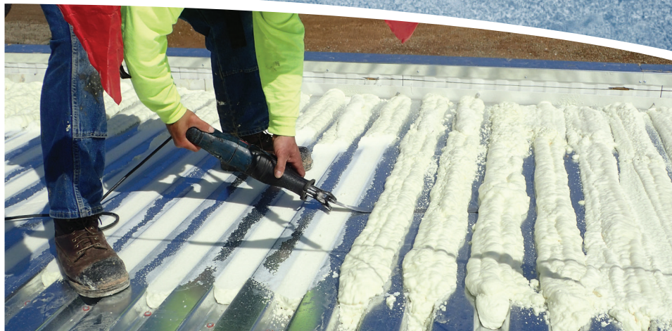
Photo 2: A view of field-installed spray foam at a roof perimeter. The worker is using a long nonserrated blade in the reciprocating saw to trim the foam flush—a laborious but necessary step.
