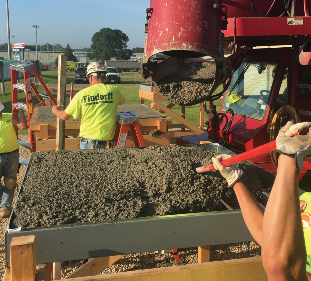
Photo 1: Exterior concrete slabs are poured by union concrete finishers. Two separate concrete loads—one normal weight structural concrete and the other lightweight structural concrete—were used.
