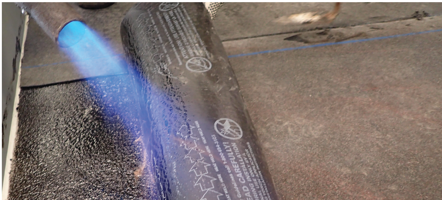
Photo 2: A view of the SBS polymer-modified bitumen base sheet being torched to a primed concrete deck during the roof system installation
