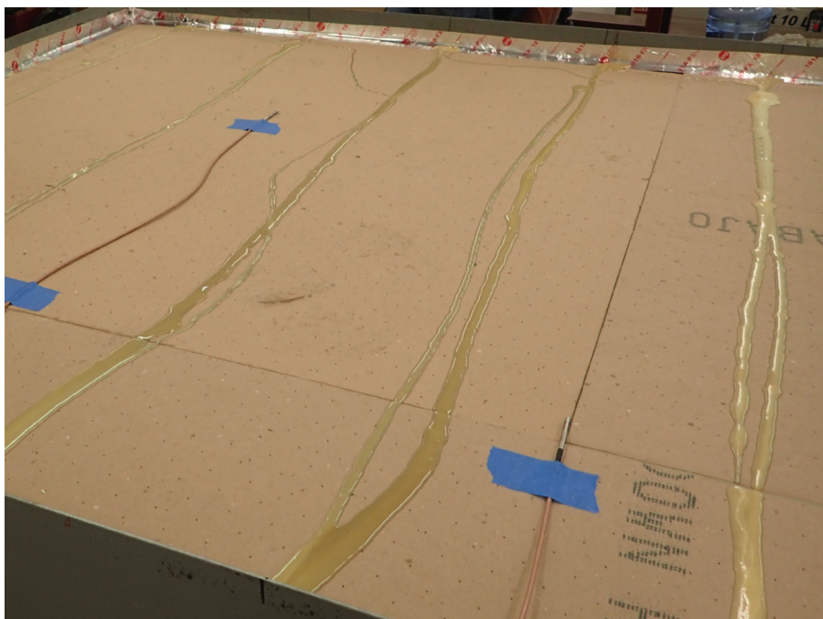
Photo 3: A view of the Phase 2 roof systems being installed over the concrete decks after 28 days. The insulation system was planned for staggered joints and installation placement of the instruments. The ribbon adhesive can be seen rising and blue tape holding the matchstick-sized temperature and humidity sensors in place.
