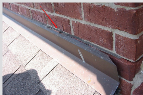
Photo 2: This saw-cut flashing is beginning to pull away from the wall, making it completely ineffective in keeping out water.
