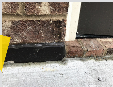
Photo 3: This concrete slab would have benefited from through-wall flashing running under the lower course of brick.
