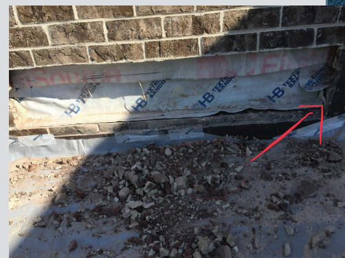
Photo 4: An example of a failure in existing through-wall flashing
