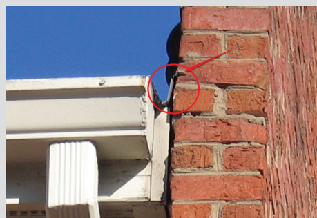
Photo 1: An example of saw-cut rather than through-wall flashing
