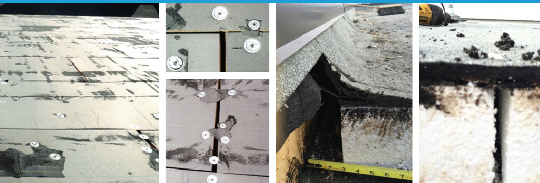
Figure 2: Typical examples of gap formations in low-slope roof assemblies. Courtesy of 2001 Company, Waterbury, Conn., and Canadian Roofing Contractors Association.
