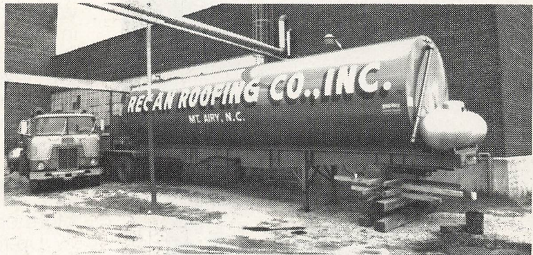
37 ton/10,000 gallon capacity
