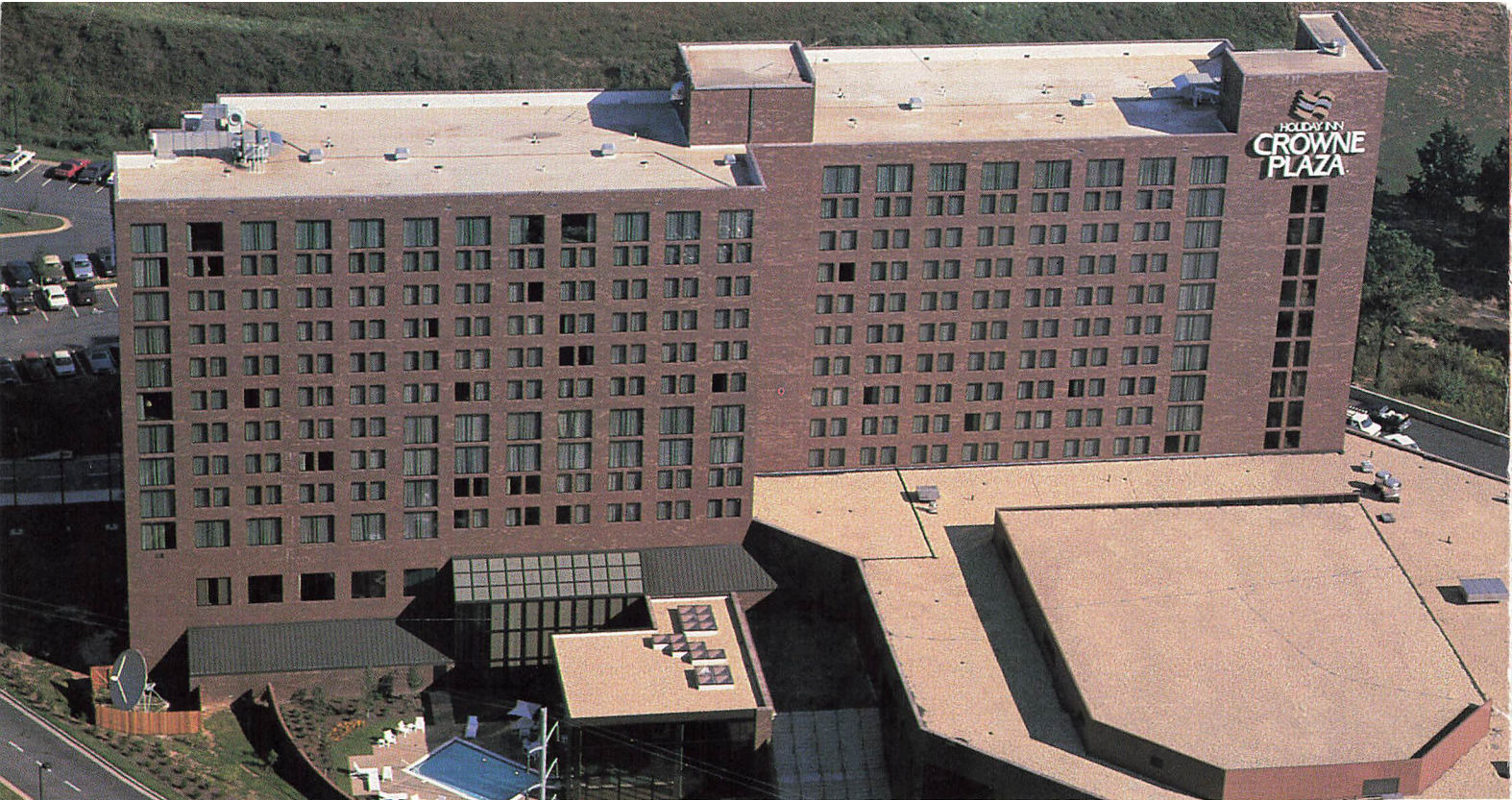
Holiday Inn/CROWNE PLAZA, Atlanta, Georgia. Southeastern States Roofing (Orlando, FL).
