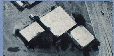
County Offices - Dallas, Texas
