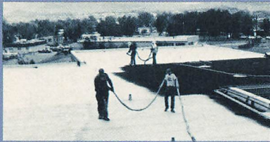
Children's Center - Thermopolis, Wyoming
