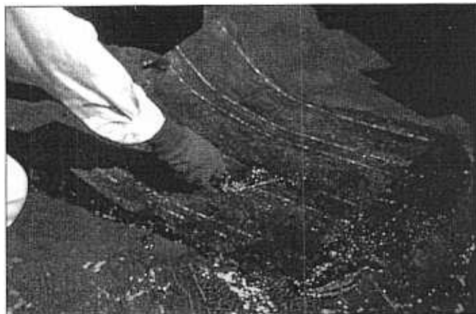
Photo 3: Setting the first patching ply in solvent-based asphalt roof cement.
