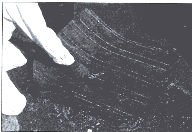
Photo 5: Installing the second patching ply to repair the previously blistered location.
