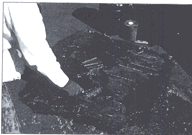
Photo 6: Applying the third layer of asphalt roof cement to the repair location.
