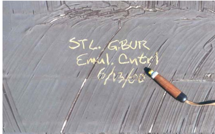
Photo 19: Depicts cracking and erosion of exposed asphalt-emulsion primer that was applied over hot asphalt glaze coat that was installed too heavy and is subsequently telegraphing, alligatoring/cracking through the overlying emulsion.
