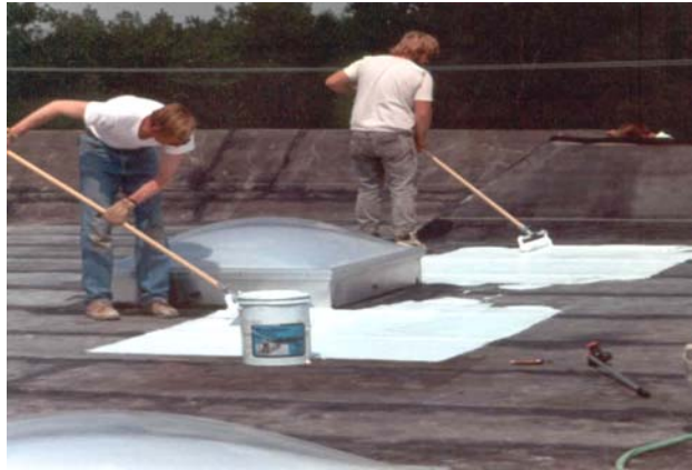
Photo 2: Application of surface coating to shield roof membrane from direct effects of weather and prolong life of roof membrane.
