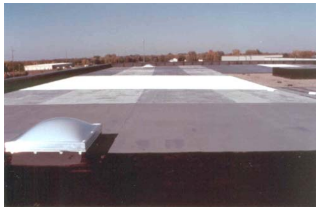
Photo 12: Depicts orientation of roof coatings applied to minimize the effects of differential thermal movement upon the coated roof membranes.
