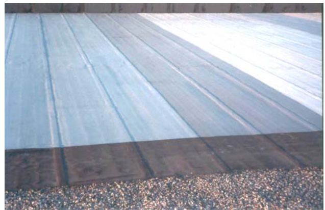
Photo 18: Overview of aluminum-pigmented, solvent-based SBS-polymer-modified and premium-grade coatings, as well as acrylic coatings that are performing well.
