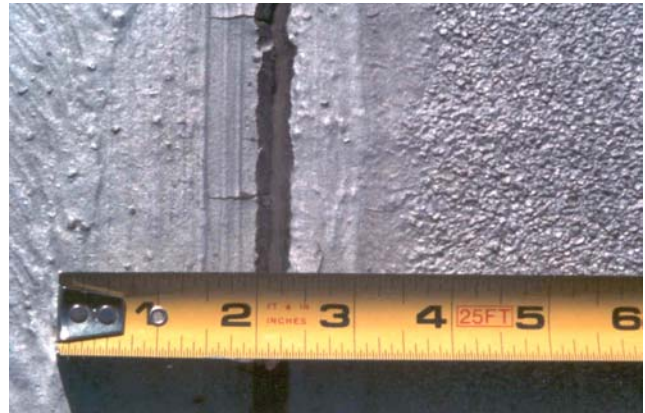
Photos 15 and 16: Stress cracks through emulsion and aluminum coating at end laps of polyester-reinforced, APP-Polymer-modified asphalt cap sheet indicates that membranes are experiencing post-application shrinkage.
