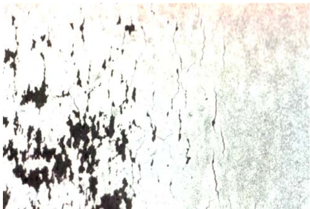
Photo 4: Shows initial cracking and peeling of surface coating.
