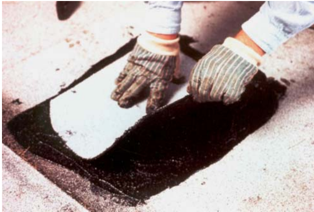
Photo 1: Shows installation of a spot repair at weather-weakened deficient location of roof membrane.
