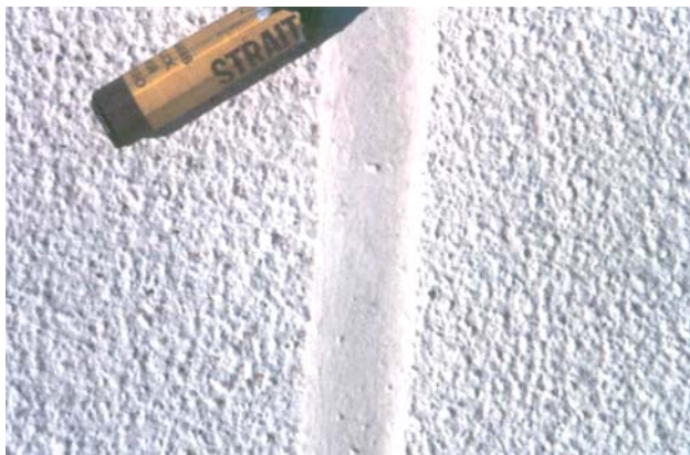
Photo 17: No stress cracks or shrinkage was evident at same SBS polymer modified asphalt cap sheet end laps coated with white acrylic coating.
