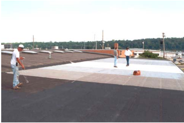
Photo 7: Shows overview of coated SBS cap sheet surfaced test roof located in Kansas City, Mo.
